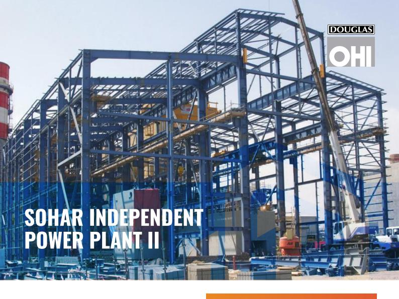
Our scope of works civil & buildings included the construction of foundations for the gas turbine generator (2 no.), steam turbine generator (1no.), transformers (2 no.) and other ancillary equipment.
