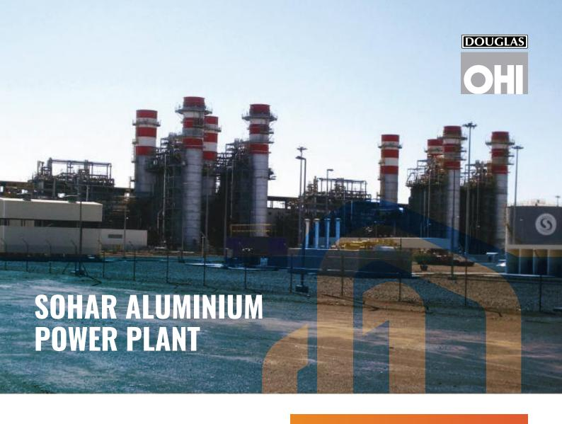
Our scope included the civil & building works for the construction of foundations for the steam turbine generator (2no.), gas turbine generator (4no.), HRSG, transformers, evaporator units, BRP pits, pump sets and storage tanks.
